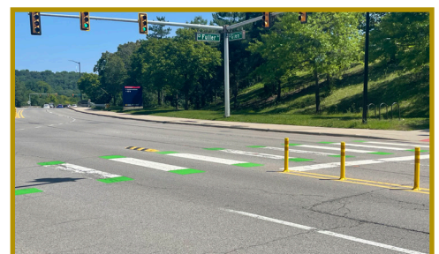
Above: Hardened centerline made of rubber speed bump and bollards. Below: Curb bump out made from bollards. Photos: Courtesy of City of Ann Arbor.
