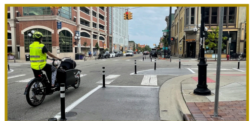
Above: Hardened centerline made of rubber speed bump and bollards. Below: Curb bump out made from bollards. Photos: Courtesy of City of Ann Arbor.
