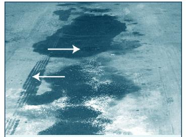
Oil and grease in direct contact with floor drain and contamination spread by moving vehicles.
