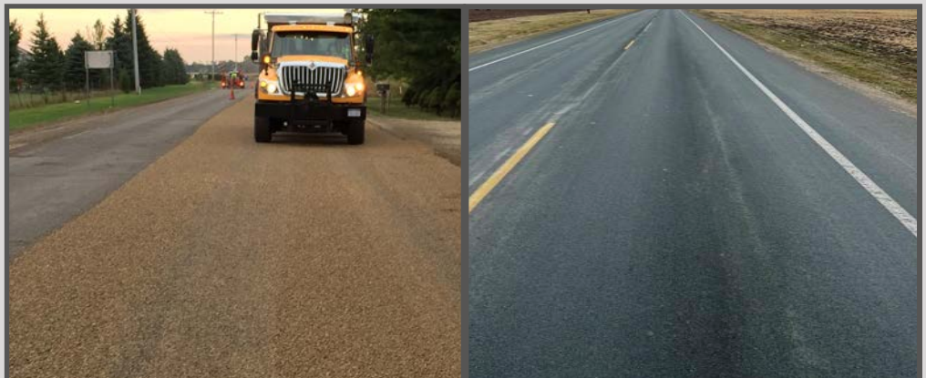
Road Commission of Kalamazoo County's Texas underseal—during Texas undersealing (left) and current (right) (photos courtesy of RCKC).
