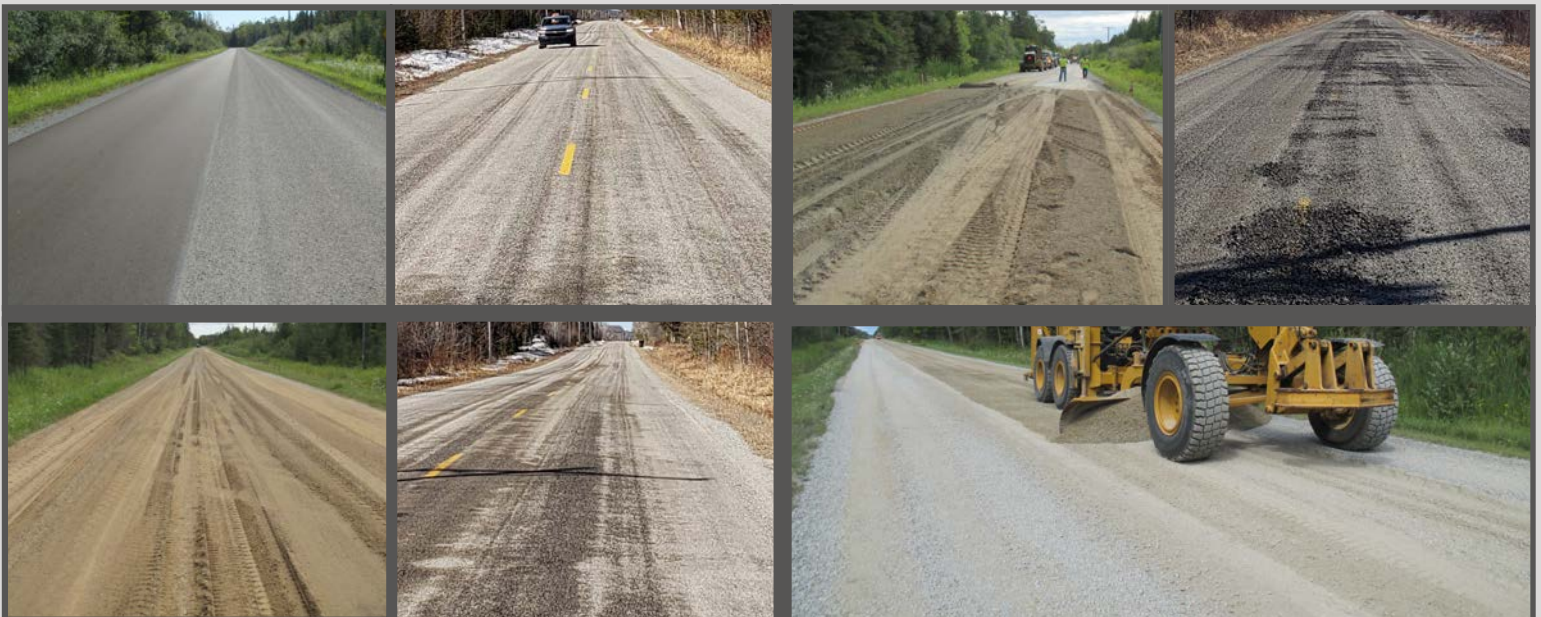
Delta County Road Commission’s gravel road stabilization test strips immediately after construction: top left—chip seal over gravel after construction (left) and the following spring (right); top right—gravel section stabilized with Perma-zyme after construction (left) and the following spring (right); bottom left—gravel section stabilized with chloride mineral brine after construction (left) and the following spring (right); bottom right—gravel section without stabilizing agent (photos courtesy of Delta CRC).
