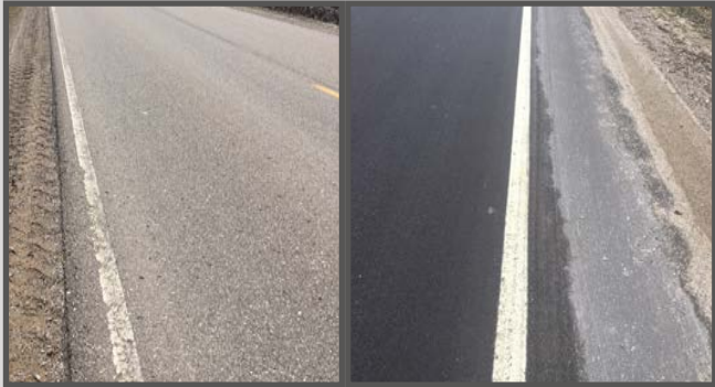
Wexford County Road Commission's Texas underseal on the M-115 detour—before (left) and after (right) (photos courtesy of Wexford CRC).
