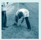
Two more sharp blows with a sledgehammer on a 3/8-inch aluminum drive rivet secures the sign post to the base.
