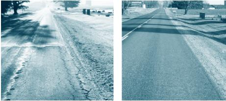
The photo on the left shows significant pavement distress, which indicates the need for heavy rehabilitation or structural improvement. The photo on the right is the same road after patching, crack sealing and a double chip seal. "Chip sealing a road that is in poor condition is like a band-aid to hold it together until we can afford to rebuild it," explained Wexford County Road Commission County Highway Engineer Karl Hanson. "It's an affordable way to buy a few more years of service."
