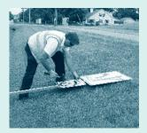
It takes two or three sharp blows with a twopound sledgehammer to fasten a sign to a post using a 3/8-inch solid aluminum drive rivet. Using an aluminum rivet prevents corrosion on the sign face caused by electrolysis and rust bleed.
