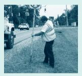
Slipping the 1 3/4-inch square, high-carbon square steel sign post into the base nearly completes the operation. The combination of high carbon steel and 3/8-inch holes every inch provides breakaway protection and meets FHWA roadside requirements. The
