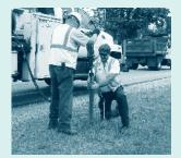
Using a truck-mounted handheld hydraulic jack-hammer, the crew drives a 36-inch long sign base into the earth. The jackhammer eliminates the need for a boom or a bucket on the truck, and also minimizes problems with overhead obstructions. The
