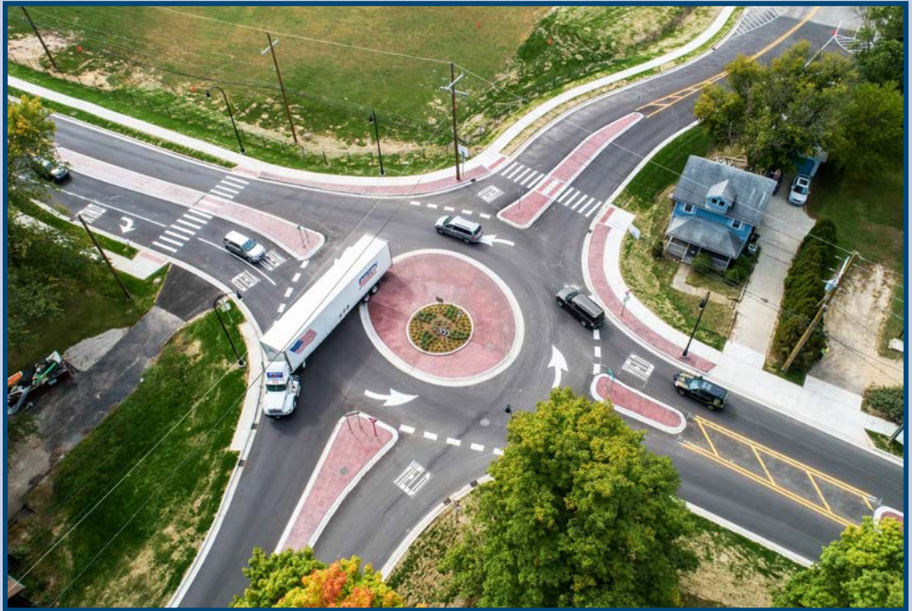
Compact roundabout at Baker-Dan Hoey intersection, City of Dexter (photo courtesy of Washtenaw CRC)
