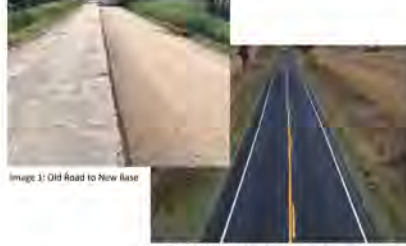
Image 2: Double Chip Seal Over Recycled Base
