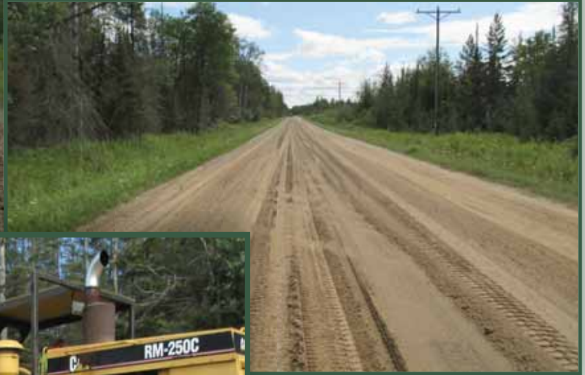
Test sections: top left – gravel section stabilized with Perma-zyme; top right – gravel section stabilized with chloride; left – reclaimer on gravel section being stabilized with Perma-zyme (Photos: CTT Archive)
