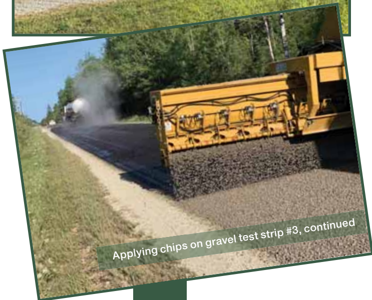
Applying chips on gravel test strip #3
