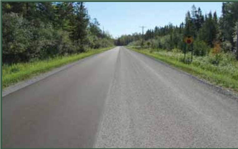
Control sections: bottom left – paved section without chipseal (left) and with chipseal (right); bottom right – gravel section without stabilizing agent (Photos: CTT Archive)
