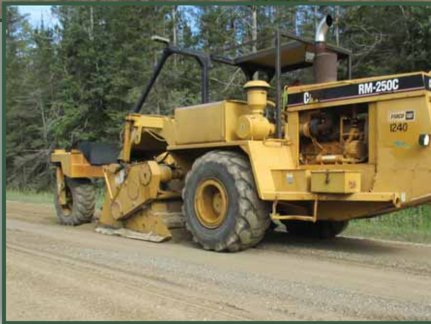
Test sections: top left – gravel section stabilized with Perma-zyme; top right – gravel section stabilized with chloride; left – reclaimer on gravel section being stabilized with Perma-zyme (Photos: CTT Archive)
