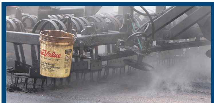
Tines scarifying the Pine Mountain Road (Photo credit: John Kiefer)
